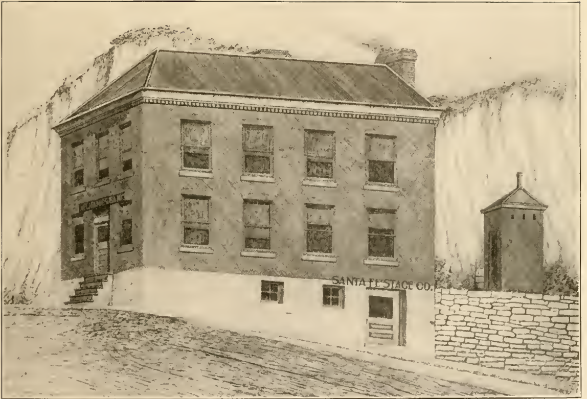
THE SANTA FE STAGE COMPANY. NORTH WEST CORNER OF SECOND AND MAIN STREETS
